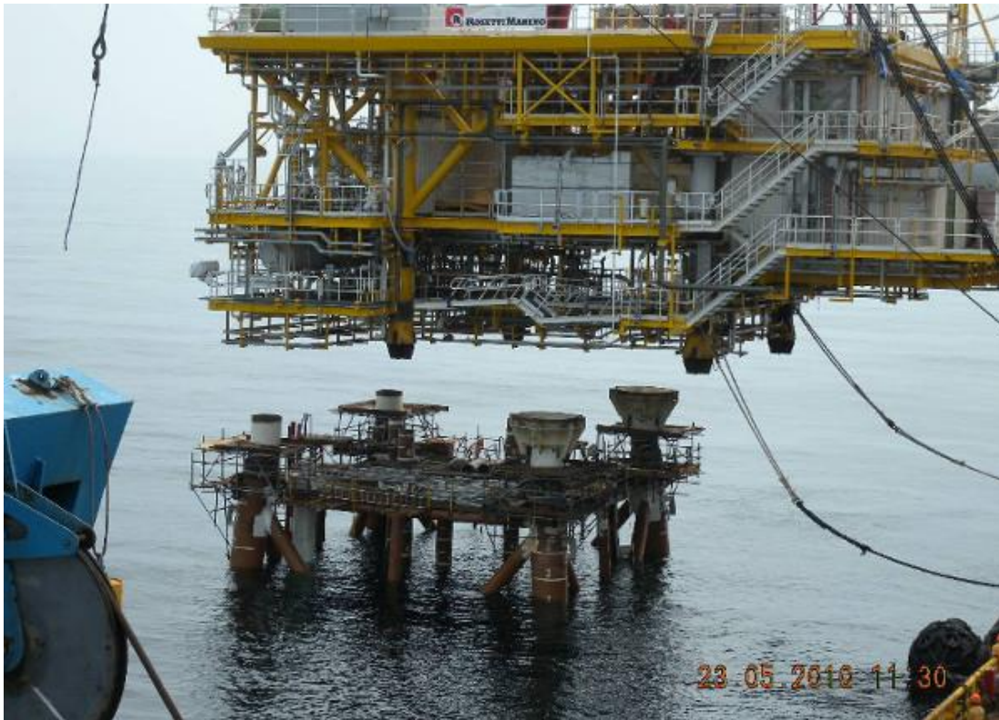
Figure 14: Platform legs and topside connection [10]
