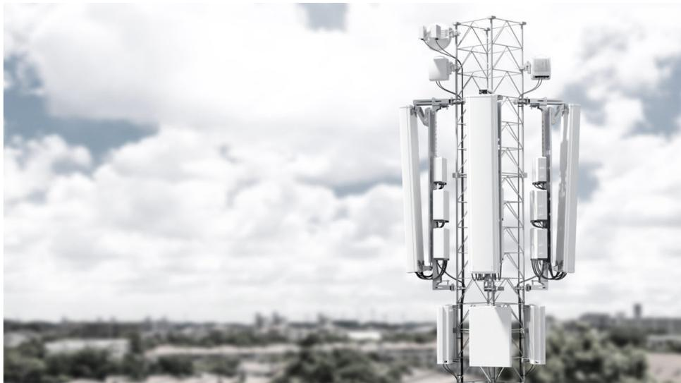
**Figure 2.1:** A 5G suburban base station (Adapted from [9])
