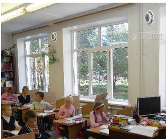
Figure 66 – Example of 2 D-MEV devices installed in a classroom.
