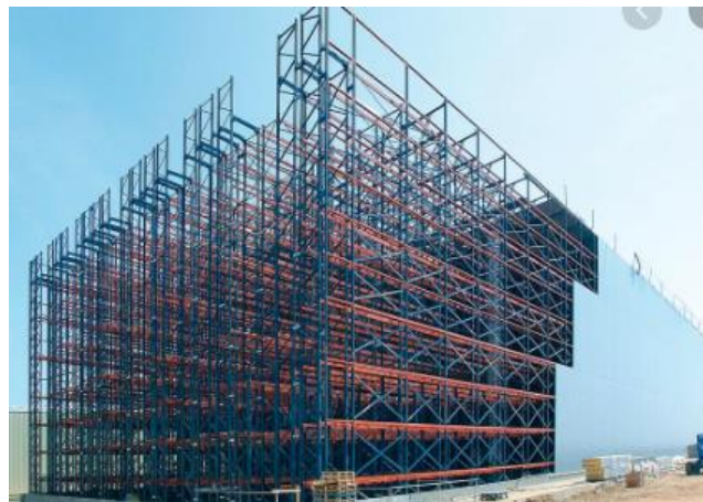
Figure 1.6. Self-supporting automated storage and retrieval system
