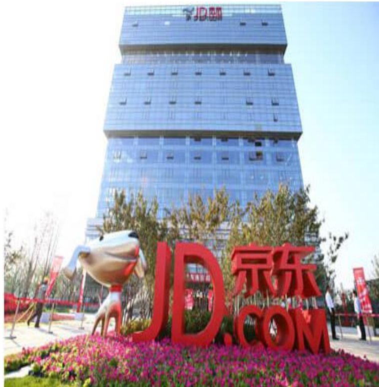
Jingdong Mall building in Beijing
