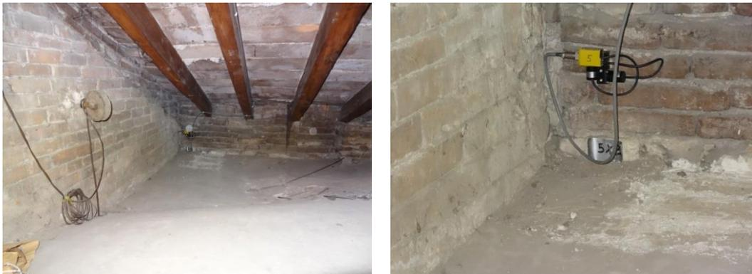
Figure 5.30- Measurement point 5 - Recording channels and accelerometers 7 and 8 [35].
