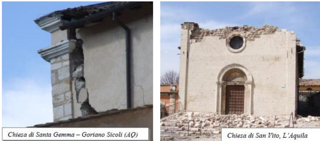
Figure 1.4 – Left: *Overturning of the façade - detachment of the facade from the walls or evident out of plumb*; Right: *Mechanisms on the top of the facade - overturning of the tympanum* [2].
