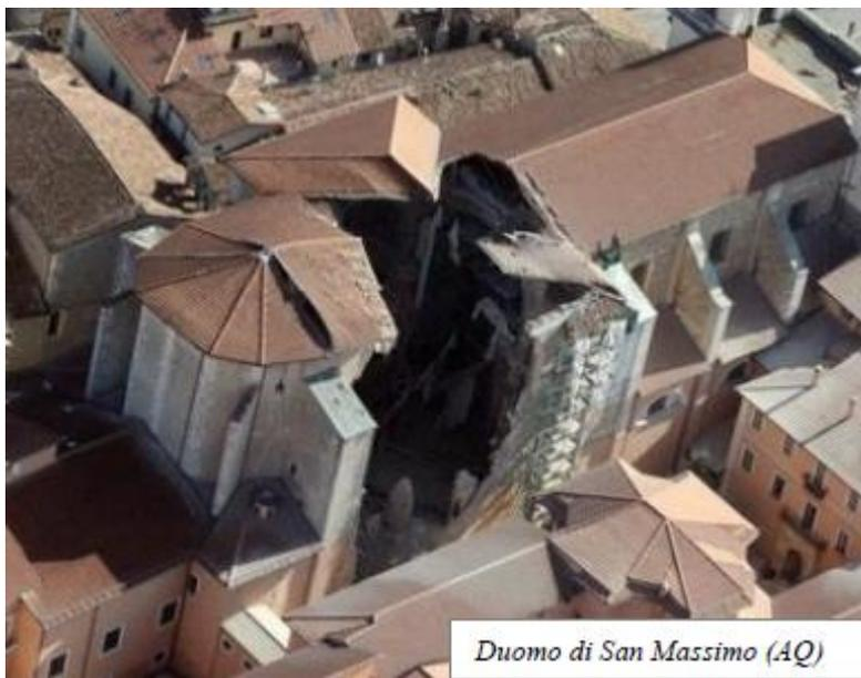
Figure 1.9 - Shear mechanisms in the walls of the transept - complete collapse [2].
