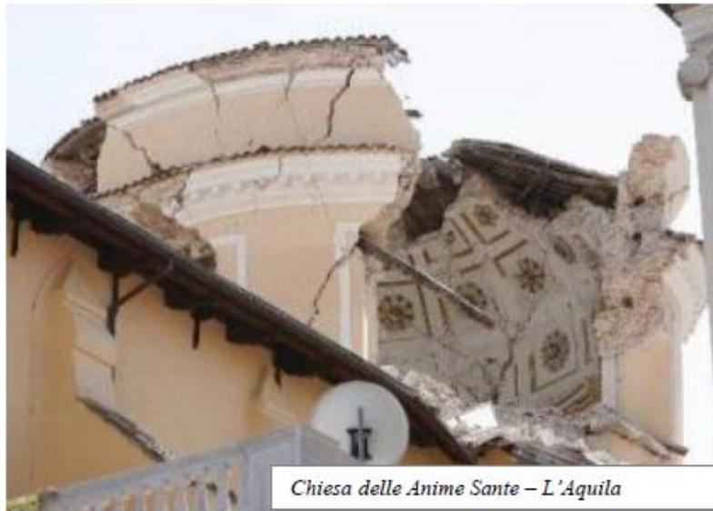
Figure 1.8 - Dome - tambour/lantern - damages in the dome with possible continuation in the tambour [2].
