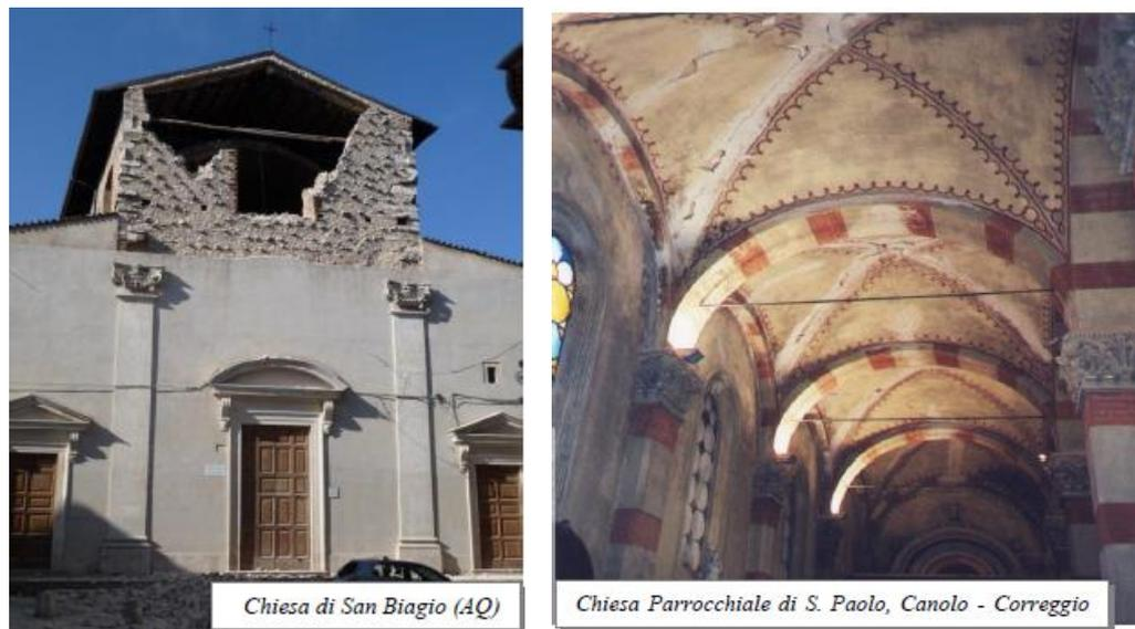
Figure 1.5 – Left: *Mechanisms on the top of the facade - overturning of the tympanum with V-shaped damage*; Right: *Vaults of the lateral naves - damage in the vaults, disconnections of the arches and of the side walls* [2].
