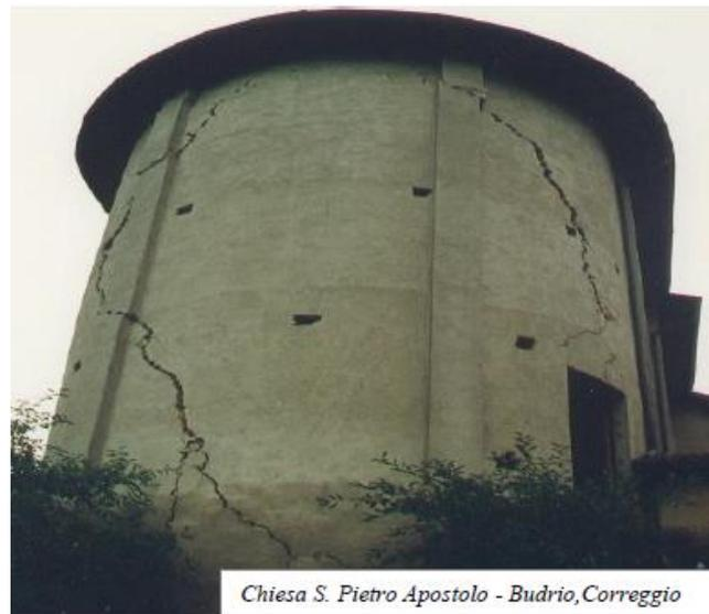
Figure 1.10 - Overturning of the apse - vertical or curved lesions in the walls of the apse [2].
