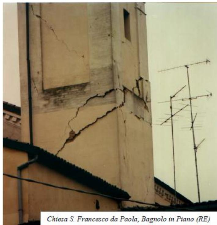
Figure 1.11 - Bell tower - damage near the detachment from the body of the church [2].
