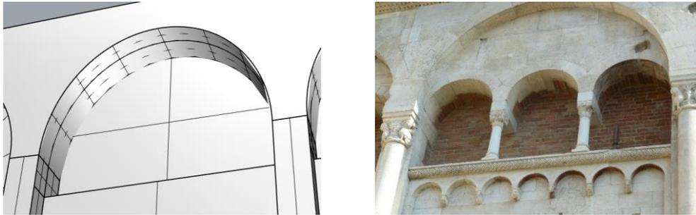
Figure 6.22 - Arches on the facade: a) 3D geometric model on Rhinoceros; b) Real detail (Google Maps Street View).
