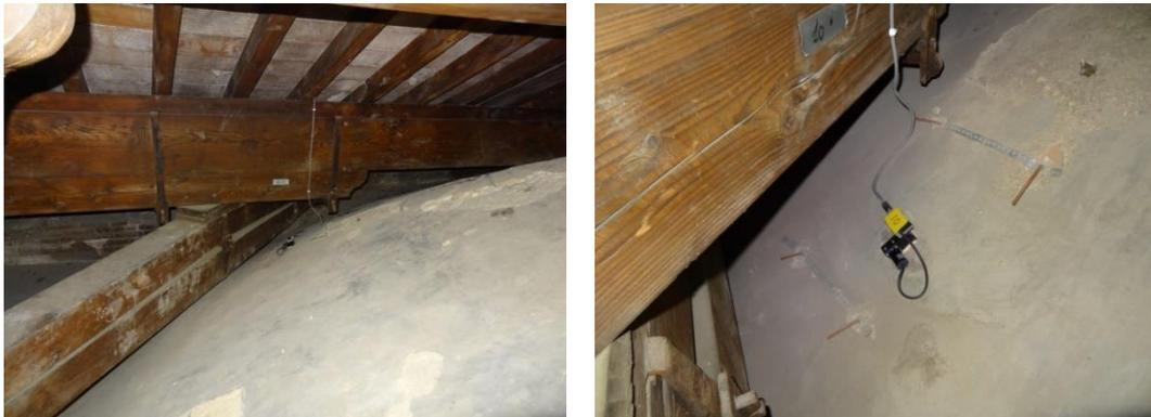
Figure 5.35 Measurement point 10 - Recording channels and accelerometers 13 [27].
