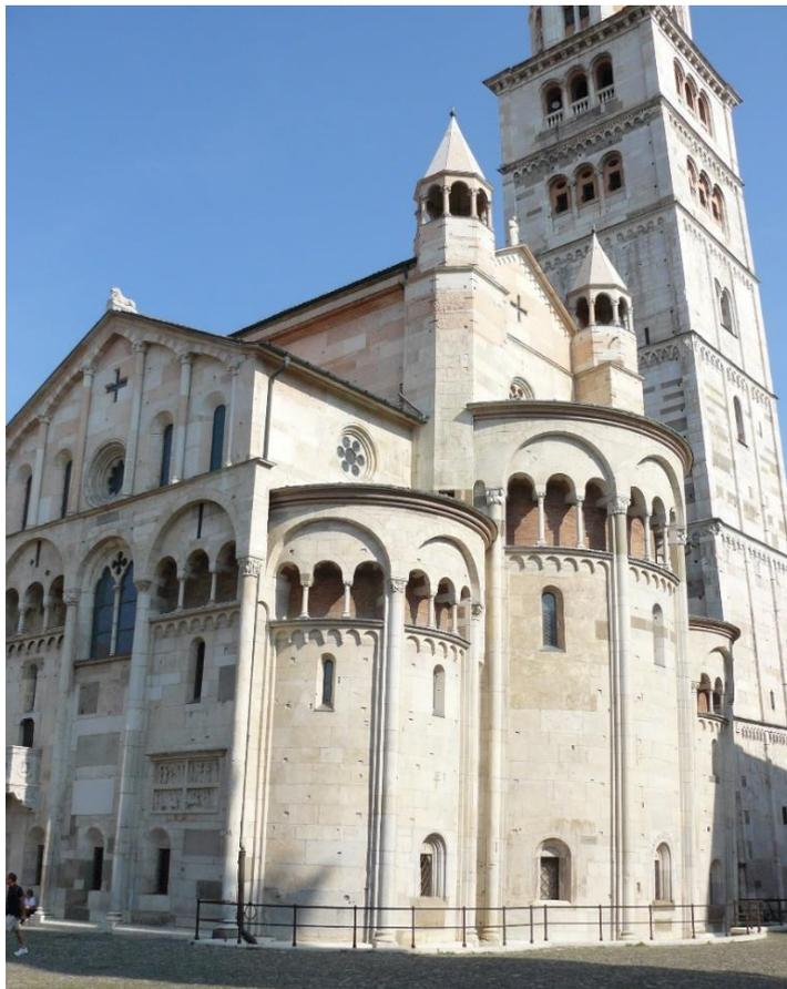
Figure 5.13 - Visible settlements in east and north directions (Photography Manuel Rovesti survey 29-08-2019).
