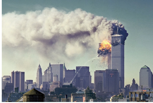
Figure 1.1: World Trade Centre twin towers collapse
