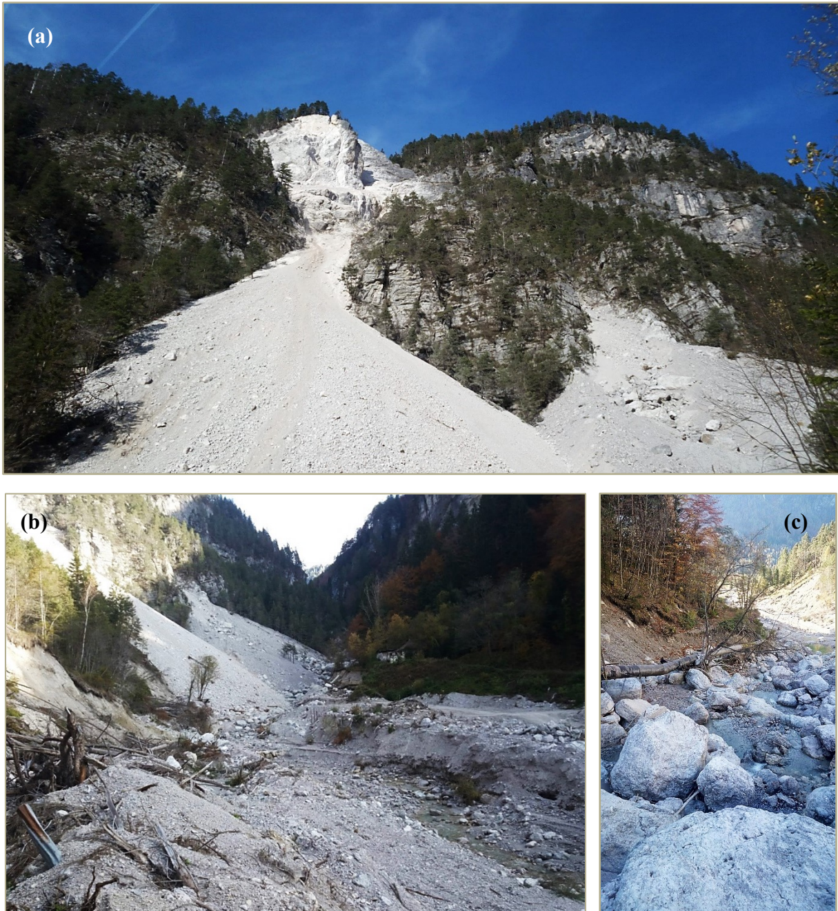
Figure 2-2 – Photographs of the site, taken during the last survey (October 24 th 2019): (a) the slope characterized by the fractured rock mass and debris deposit, (b) the torrent along the valley and (c) the blocks accumulated over the upper portion of the torrent.
