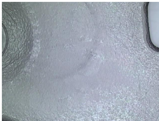
Figure 4.10. OGP inspection of Solo Smart retainer shelf, 2900 PSI
