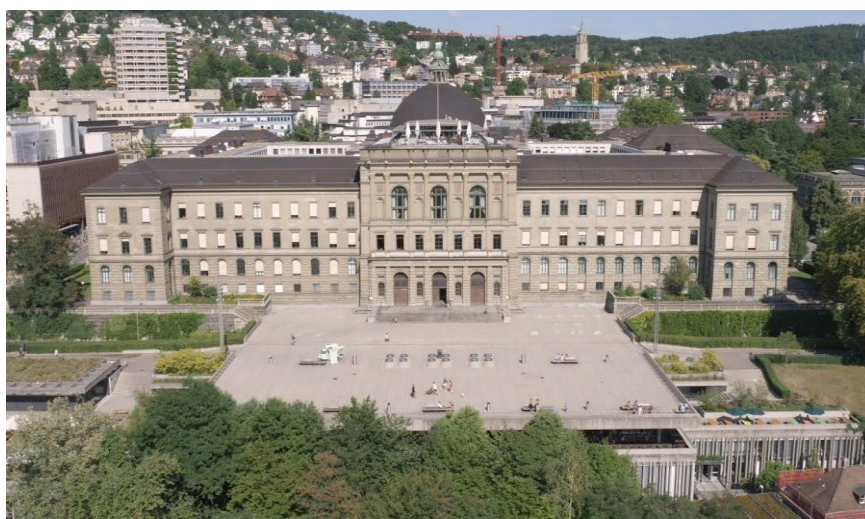
(Figura 5) 2018, ETH, Vista aerea, ethz.ch/de/campus.html
