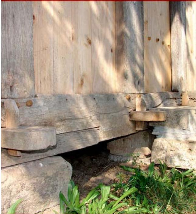
Figure 52. The structure of mortise and tenon appearing in ancient French buildings (Mortise and Tenon joints - Penchard, 2018)
