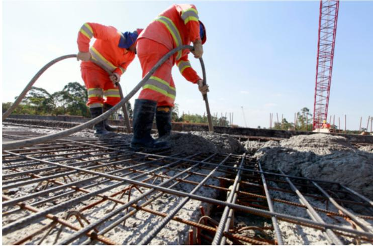
**Figure 1.16** On site pouring concrete. Figure taken from “Calcestruzzo Armato”, Teknoring.com.
