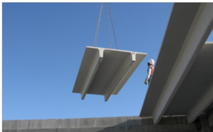
**Figure 1.15** Prefabricated module. Figure taken from “TT Beam”, Viprocosa.com.
