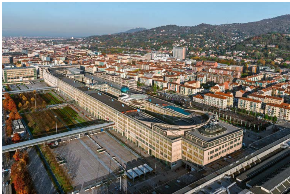
Figure 53 The Lingotto factory was a striking modern architecture for its time. For its reinforced concrete structure and the use of functionalism in production, Le Corbusier took it as an inspiration for his studies.
