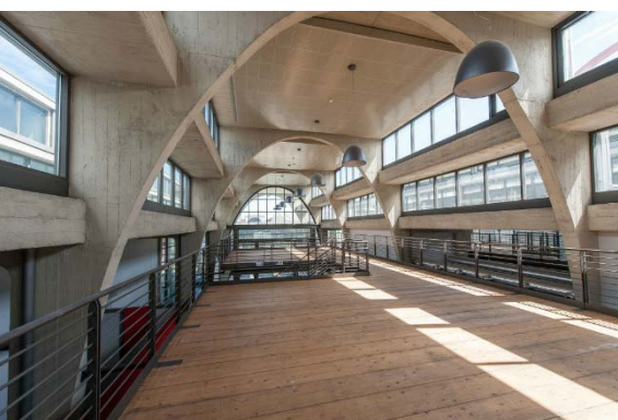
Figure 26 The interventions inside the galleries: internal space division (above), and addition of demountable mezzanine floors (bottom).
