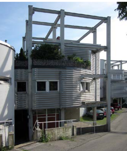
Figure 46 The complex structural system of the Wohnbau Neufeldweg would allow deep modification of the building itself.
