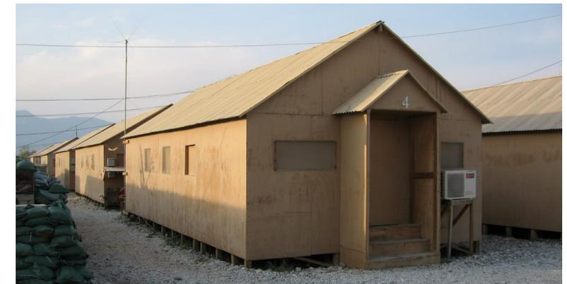
Fig. 83: Barracks Hut in legno compensato, Afghanistan, 2003 (a destra).
