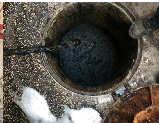
Figure 67. Leakage of waste water in telecom manholes
