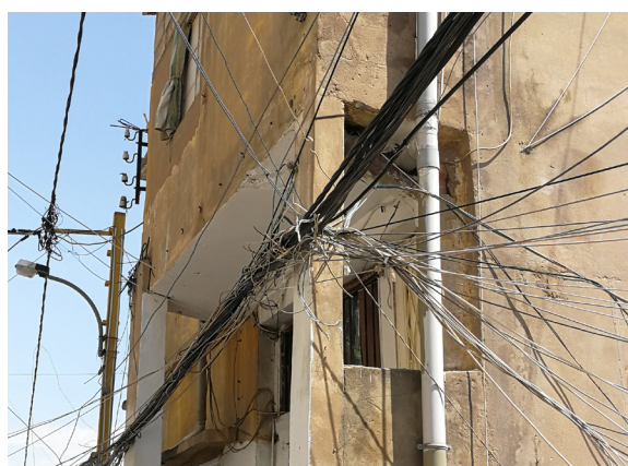
Figure 64. Tangled Hazardous Wires
