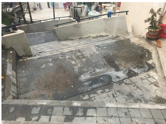
Figure 66. Blocked Drains and malfunctioning Sewage
