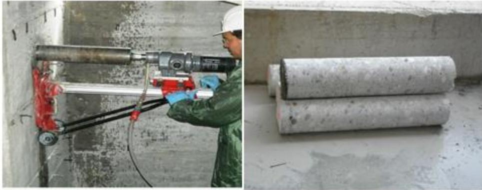
**Figure 3.8 Concrete samples taken by coring**
