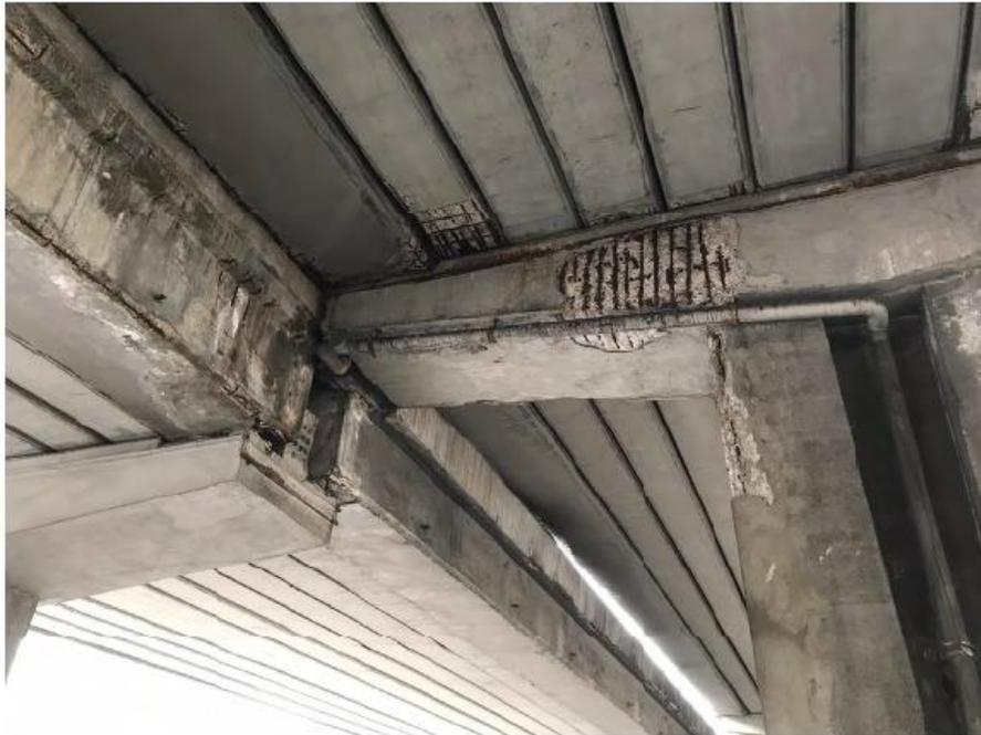
**Figure 2.2 Example of degradation due to corrosion [16]**
