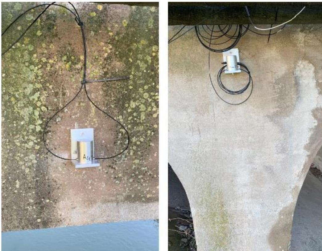
Figure 3.49 Accelerometer 1 and accelerometer 3 on the left side of the bridge
