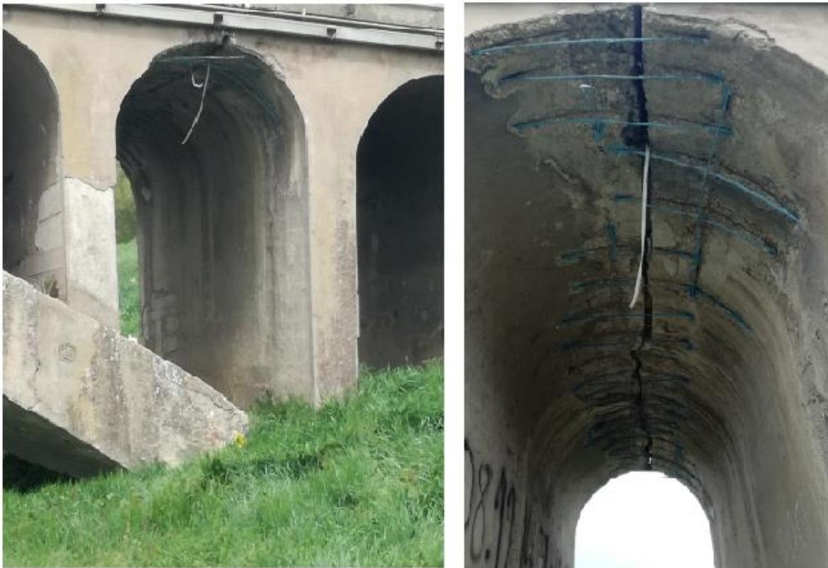
*Figure 3.39 Condition of the third arch opposite to the center of Cannara during inspections*
