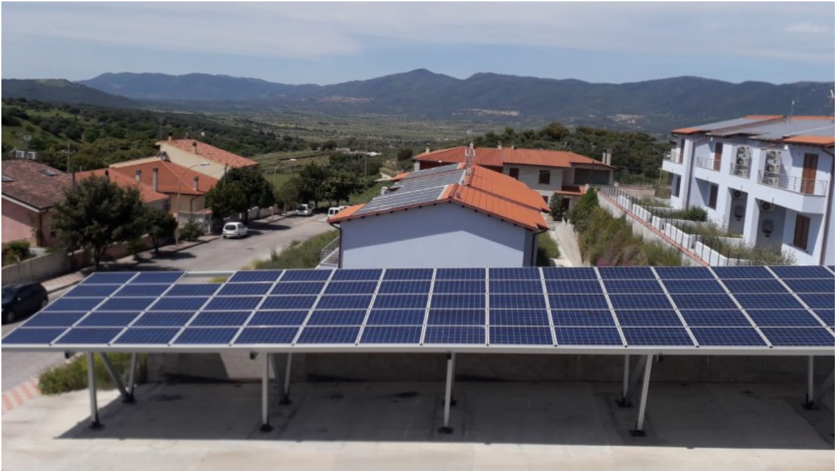
Figure 4: shared PV installation feeding the municipality of Benetutti.
