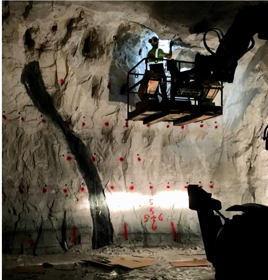
Figure III.6 Charging of the roof holes
