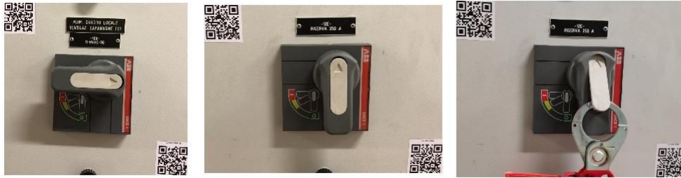
Figure 2.10. Examples of photos in the first dataset. From left to right it is possible see the switch in the state: on, off, extract.
