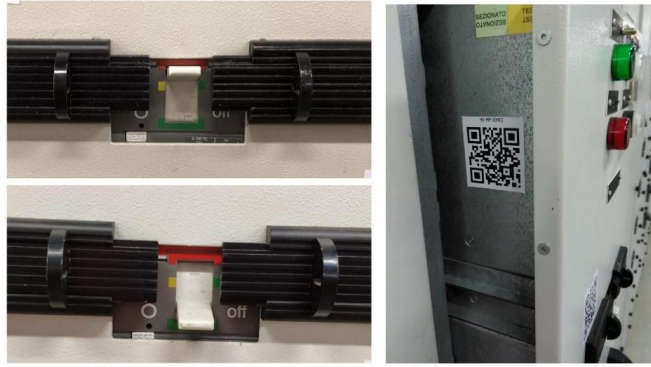
Figure 2.11. Examples of photos in the second dataset. On the left, the top photo shows when the switch is on while the bottom one shows when it is off. On the right an image of when the switch is extracted.
