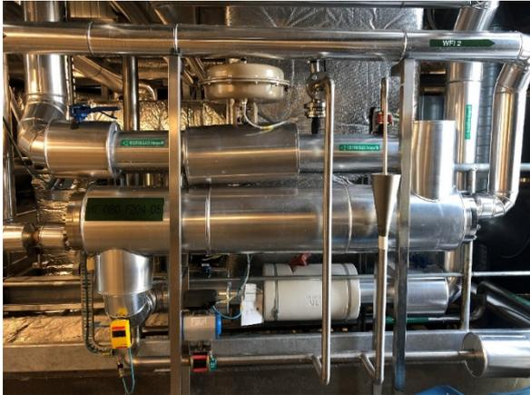
Figura 37: Scambiatore shell and tube WFI
