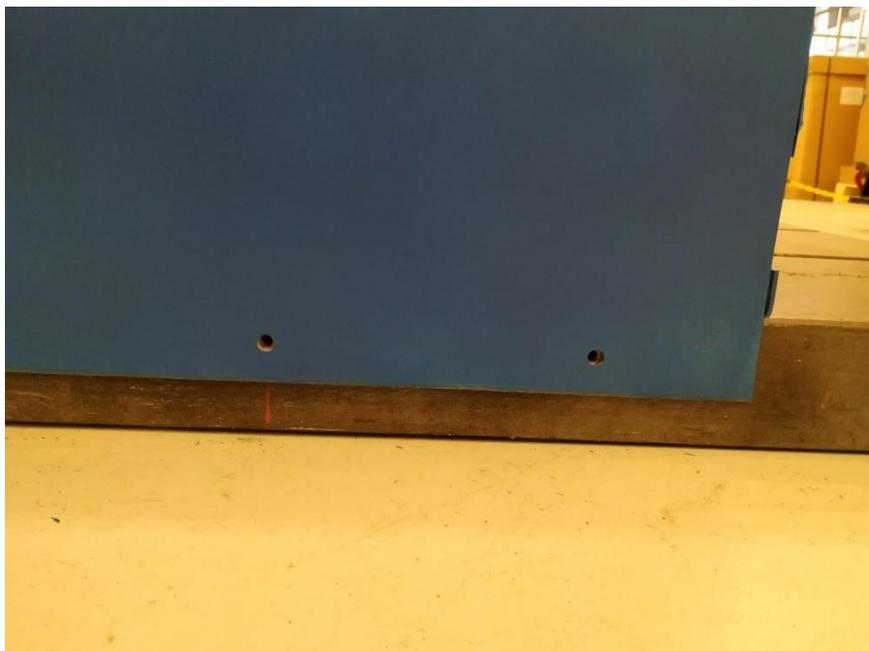
*FIGURE 85 - Holes of the barrier that does not coincide with the hole of the station in the lower part*
