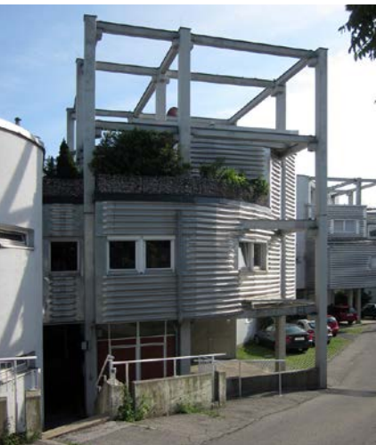
Figure 1.46 The complex structural system of the Wohnbau Neufeldweg would allow deep modification of the building itself.
