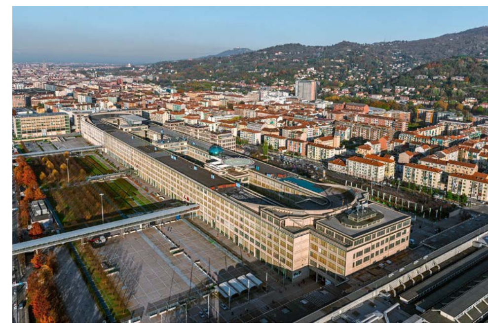
Figure 1.52 The Lingotto factory was a striking modern architecture for its time. For its reinforced concrete structure and the use of functionalism in production, Le Corbusier took it as an inspiration for his studies.
