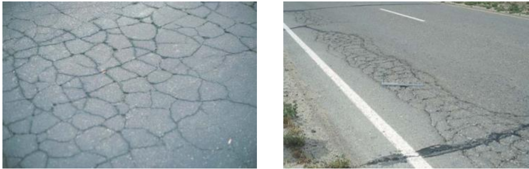
Figure 2.14: Fatigue cracks of flexible pavement
