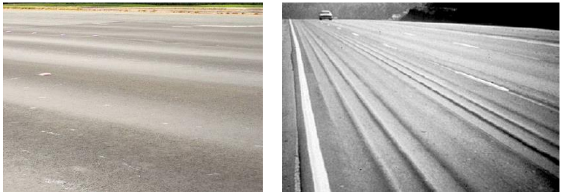
Figure 2.15: Permanent deformation in flexible pavement
