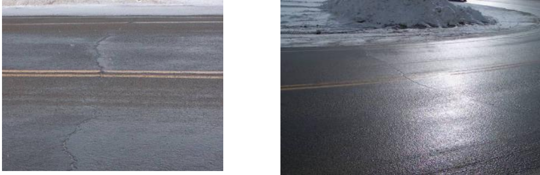
Figure 2.16: Transversal thermal cracks in flexible pavement
