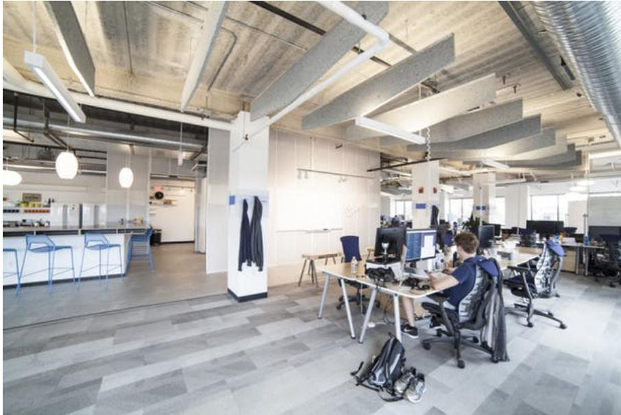
*Fig. 8: Example of applications of baffles on ceiling.*
