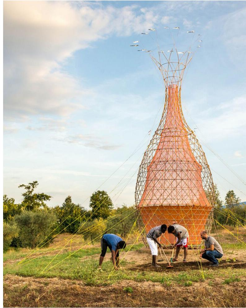
“Warka Water relies only on natural phenomena such as gravity, condensation & evaporation and doesn’t require electrical power. It is a vertical structure designed to harvest potable water from the atmosphere (it collects rain, harvests fog and dew). Warka Water is designed to be owned and operated by the villagers, a key factor that will facilitate the success of the project. The tower not only provides a fundamental resource for life – water – but also creates a social place
