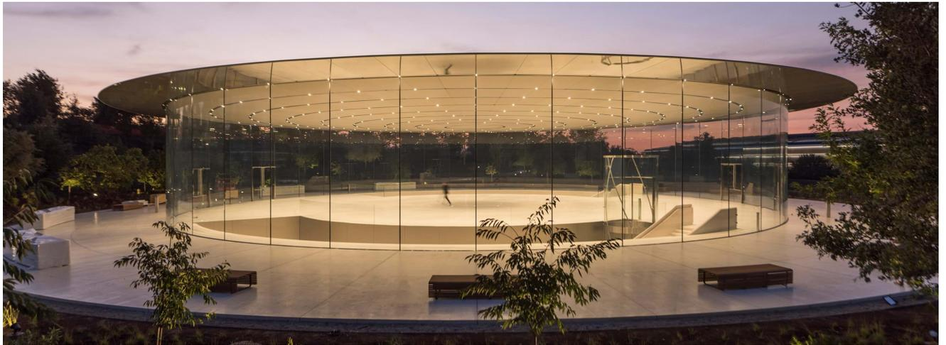
carbon-fiber roof in the world, it weighs 80.7 tons (73.2 metric tons), with just four layers of glass forming the structural support. It comprises 44 identical radial panels, which were assembled on-site and carefully craned into position onto the completed glass cylinder in a single lift. All its services, such as electric conduits and sprinkler pipes, are invisibly integrated within the thin silicone joints between the curved glass panels.”
