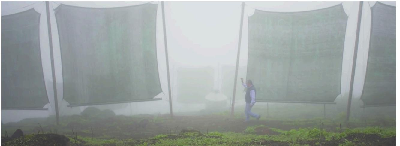
of water. The nets are set up along the foggy areas of coastal Peru and are connected to pipes, which collect the water for larger storage tanks. Residents can then use this water as irrigation for crops or to raise animals. And while the water isn't currently drinkable, Gutiérrez is working on a solution to that as well."
