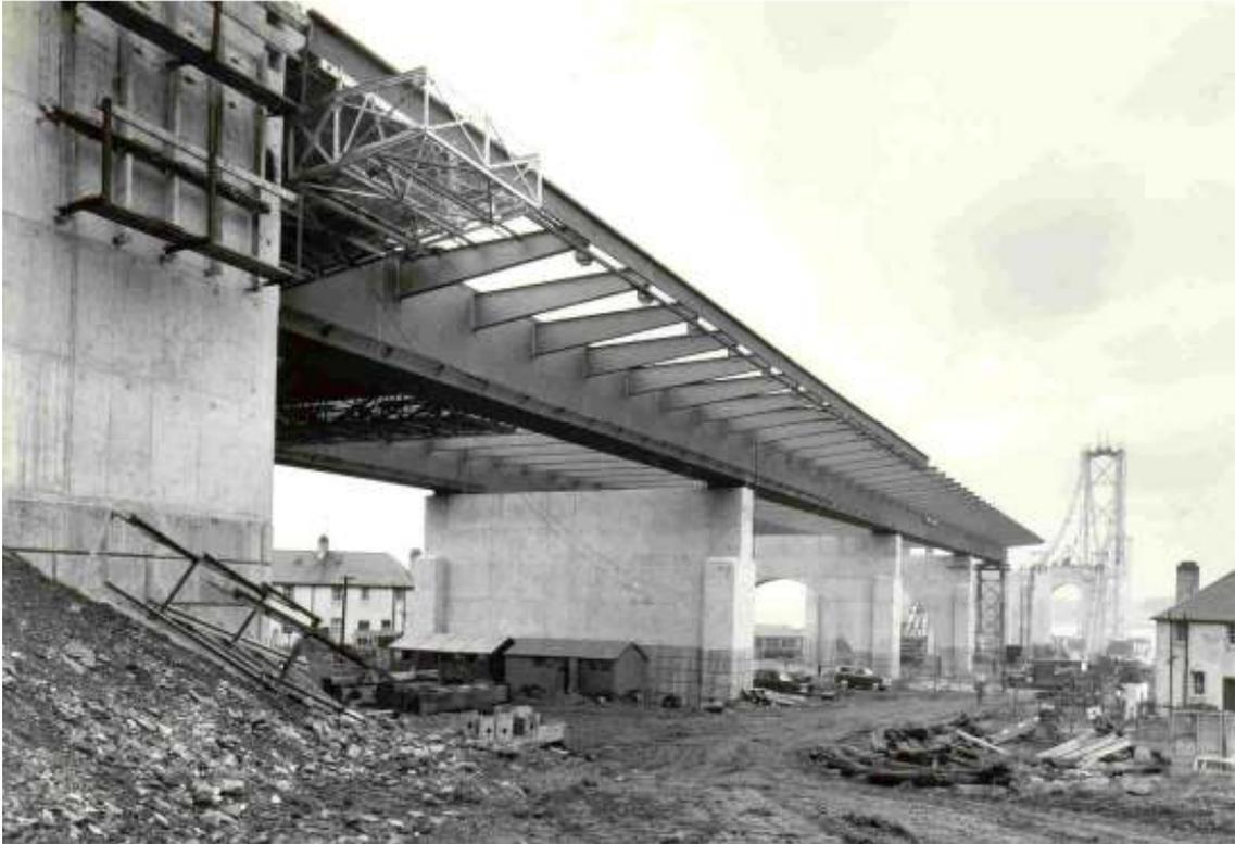
*Figure 2.4: Construction of the deck on the south viaduct (Transport of Scotland, 1964)*
