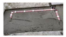
Figure 6.1: Road embeddment of the 9 turns WPT in dry concrete.
