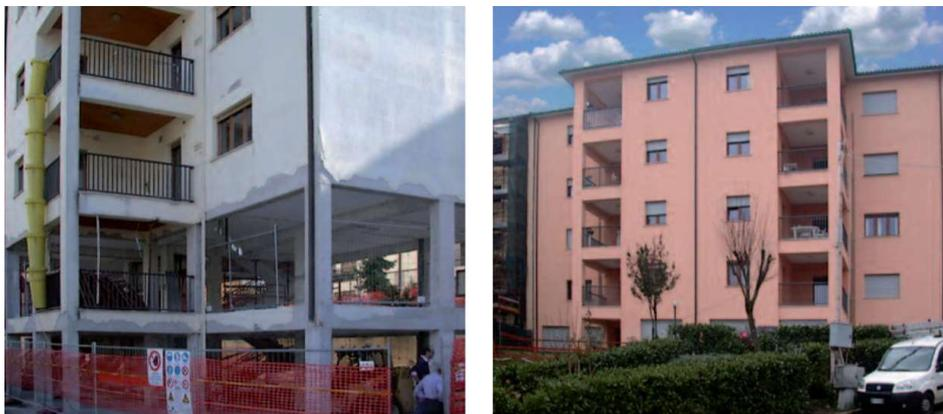
Figure 2.26 Apartment block G4, via Beffi, Coppito, before and after the intervention of seismic adaptation
