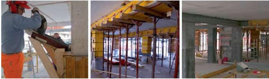
Figure 2.25 - Casting phases of seismic retrofit intervention with UHP-FRCC
