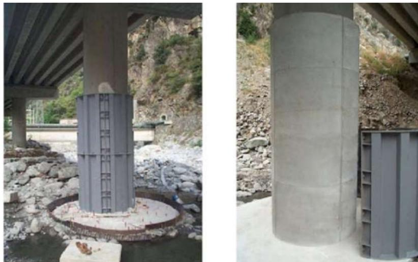
Figure 2.28 Repair and protection of foundations and supports of the Valabres viaduct
