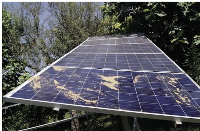
*Figure 4.4 Example of soiling*
