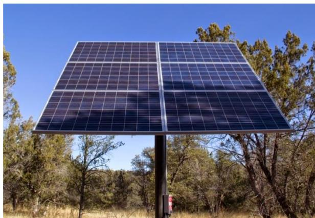
*Figure 4.9 Example of shadowing*
