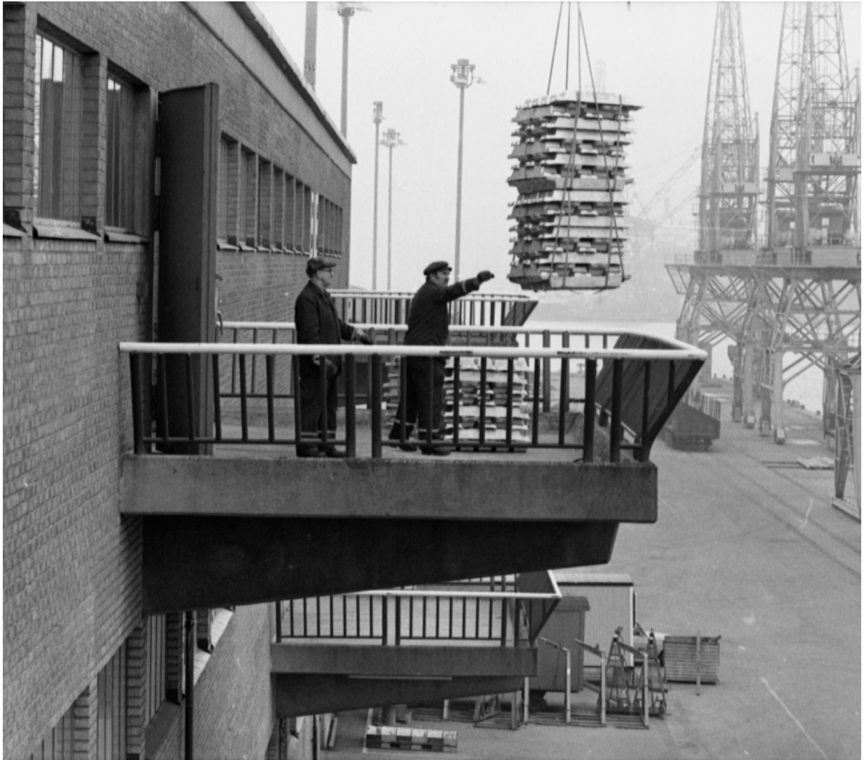
Im. 4.III.1: "Metal pallets landing on the balcony of the Magasin 113 in the Frihamnen, 1979". Taken from: http://alvstaden.goteborg.se/vara-delomraden/frihamnen/
