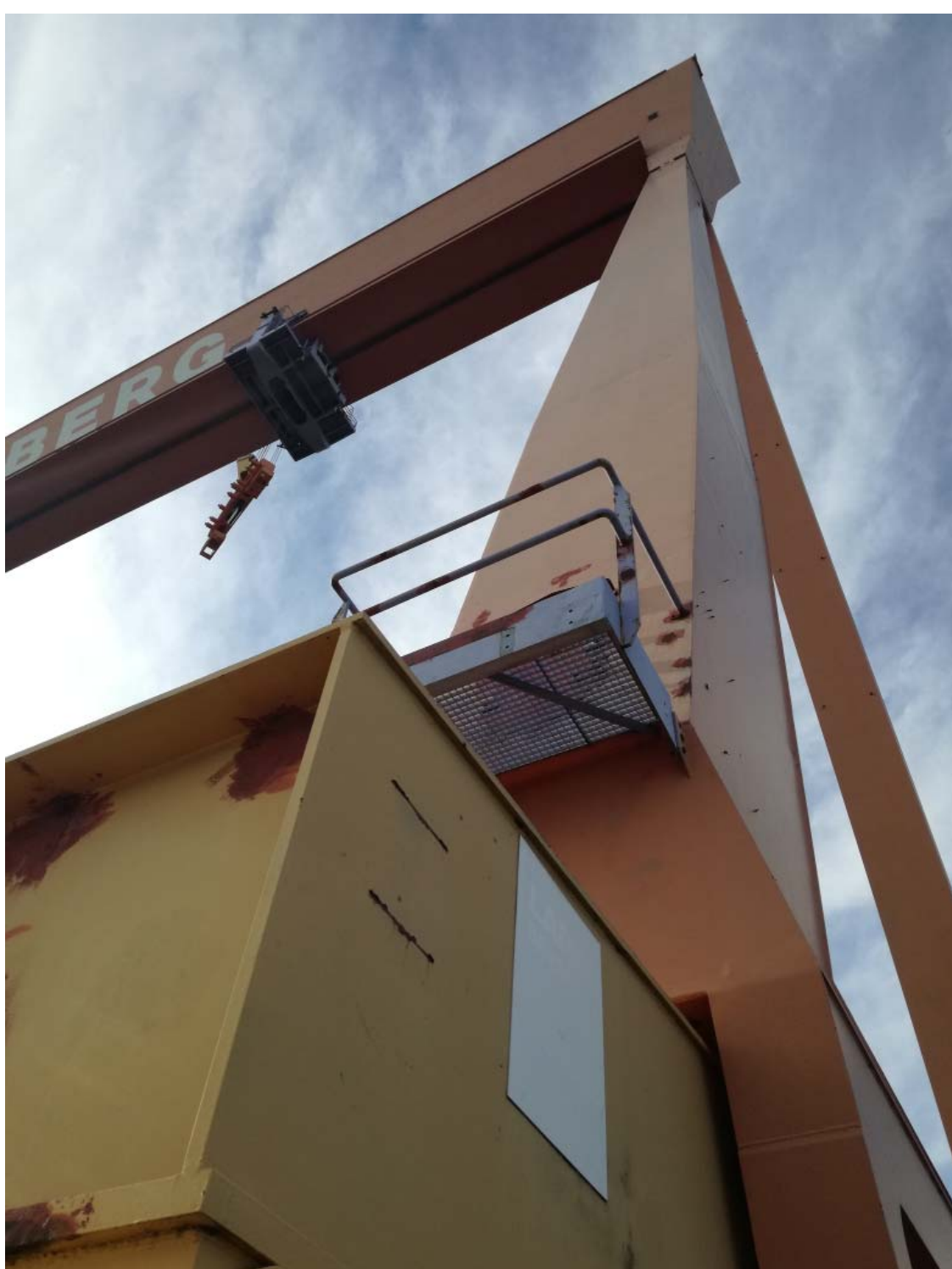
Im. 3.III. 28: Detail of Eriksberg crane. An old structure from the shipbuilding past seemed to me like a triumphal arch of the area that showed its own past with pride.
