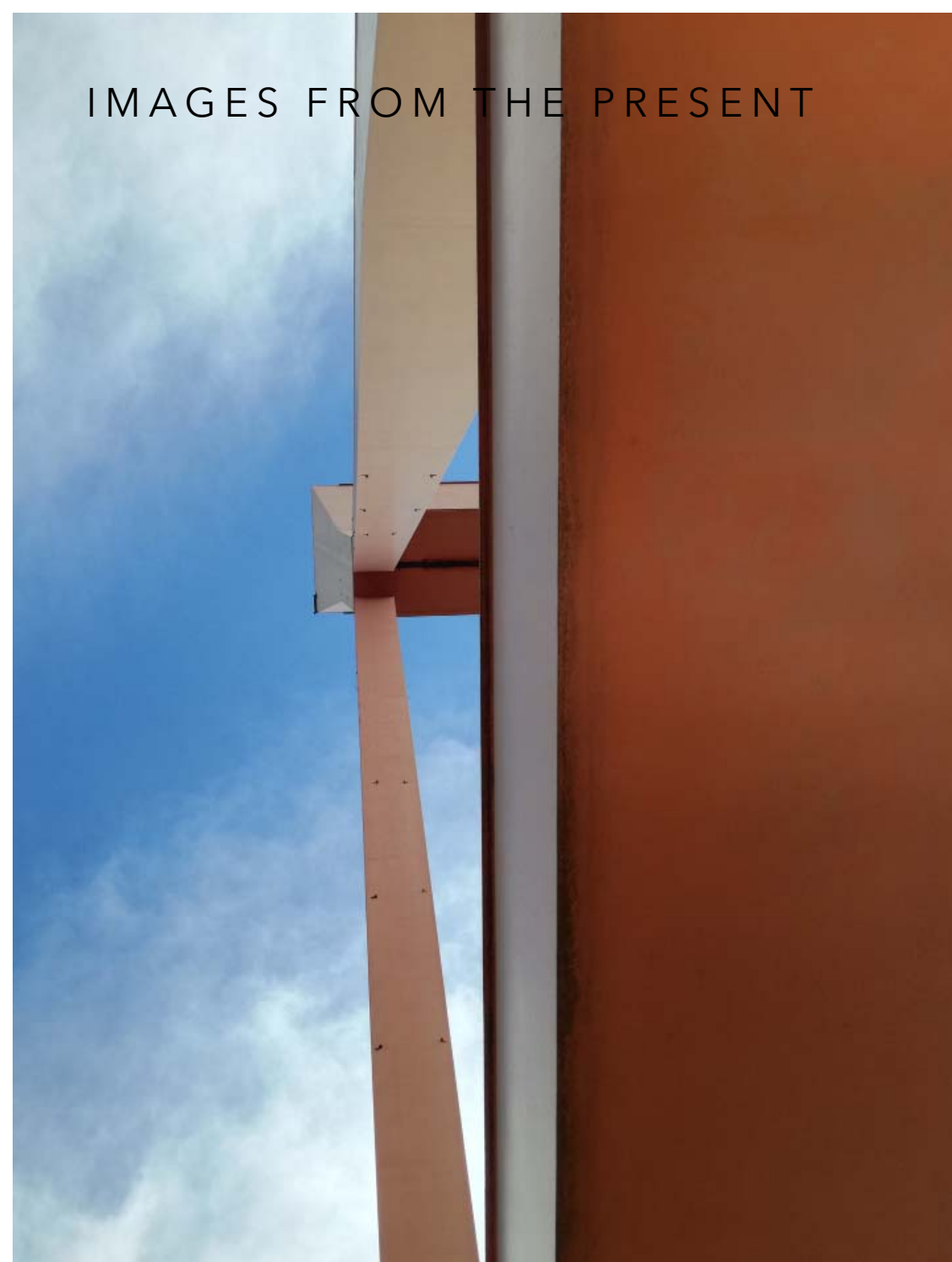
Im. 3.III. 27: Detail of Eriksberg crane.
