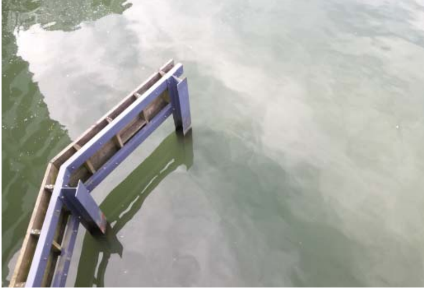
Im. 3.III. 29: Detail of water with an old structure.
