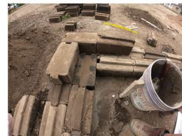
Picture 10. Interlocking bricks at corner, inside angle . Source: photo by Author.
