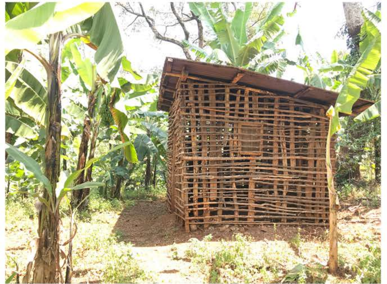
Picture 01. Structure of walls made from wooden sticks in Shimbwe. Source: Photo by the Author.
