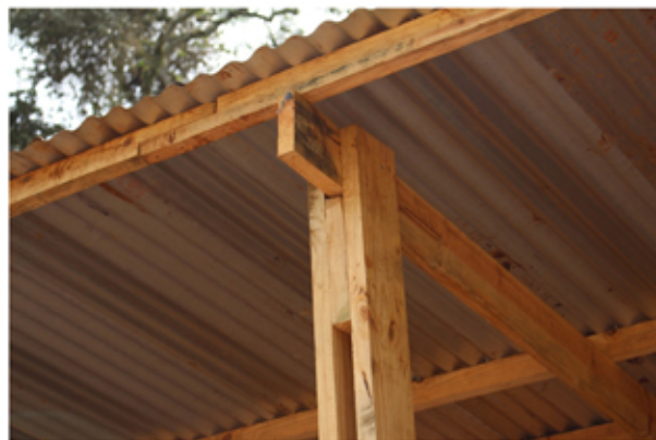
Picture 27. Wooden joint in roof. Source: Photo by the Author.
