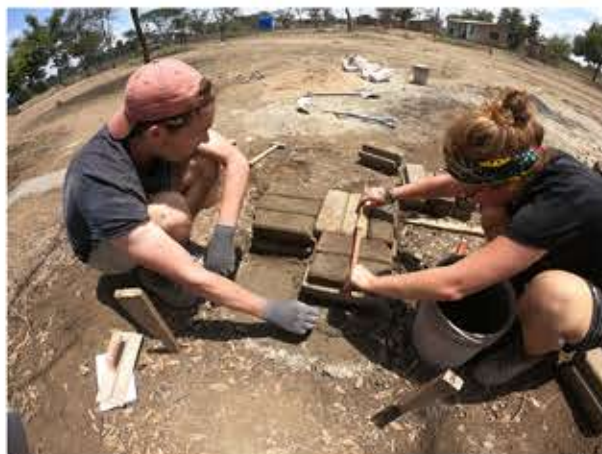
Picture 11. Levelling bricks. Source: Photo by the Author.
