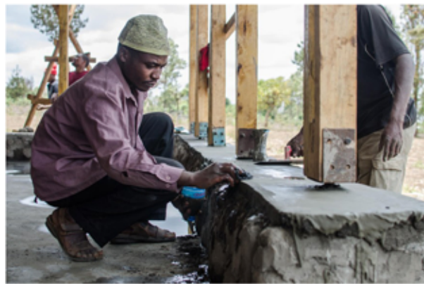
Picture 26. Tanzanian worker cleaning mortar leveling. Source: Photo by the Author.
