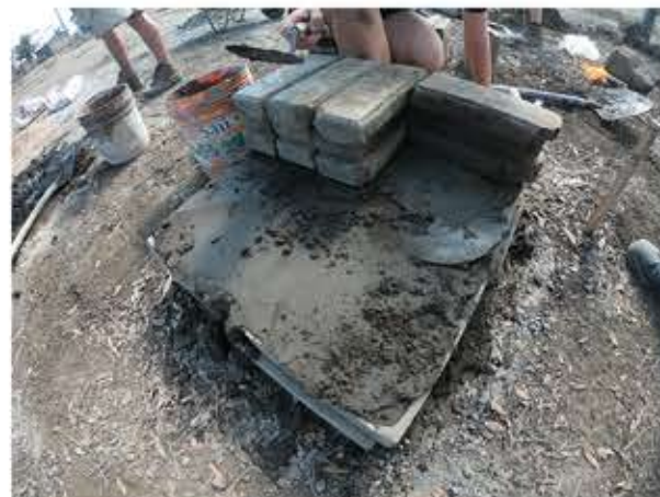
Picture 12. Mortar between bricks. Source: Photo by the Author.
