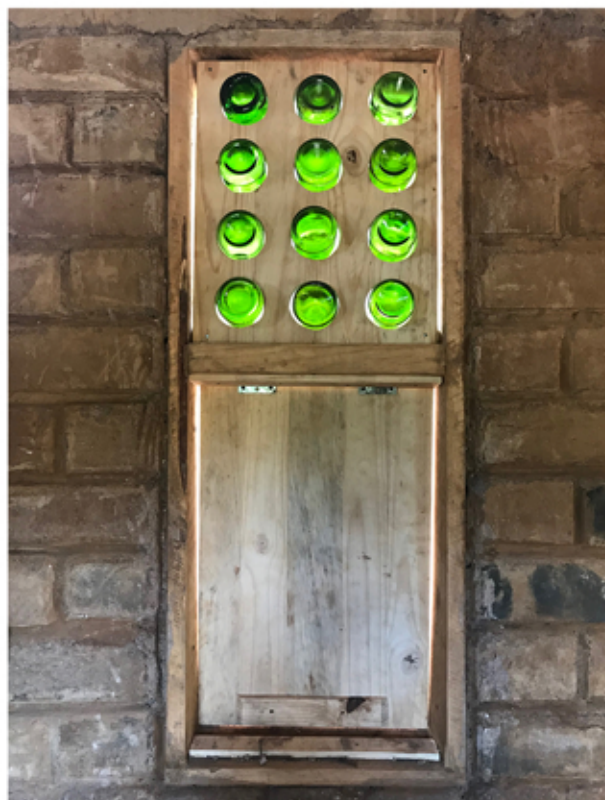
Picture 21. Front view of window prototype, developed with C-re-aid NGO, made from recycled wine bottles in wood frame. Source: Photo by the Author.
