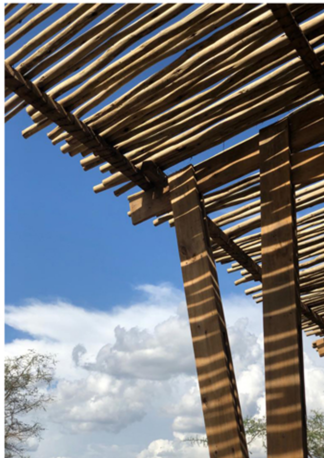
Picture 28. Wooden joints for roof sticks. Source: Photo by the Author.
