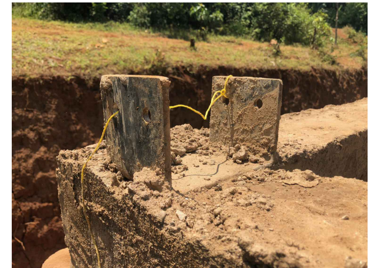
Steel foot installed in the ring beam
