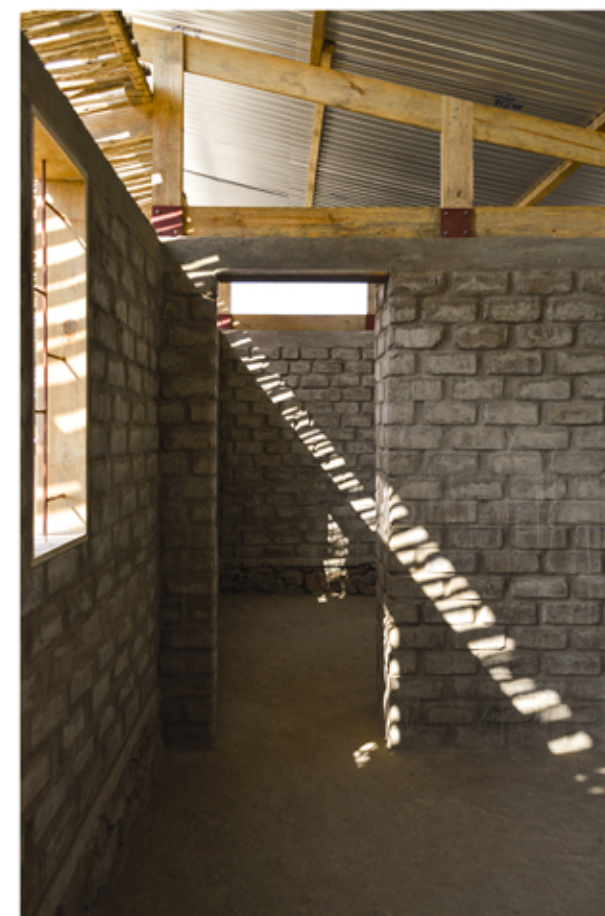
Picture 30. Interior of Doctor's house in Maji Moto portraying wooden beam structure for corrugated iron sheets. Source: Photo by Studio totale Firenze.
