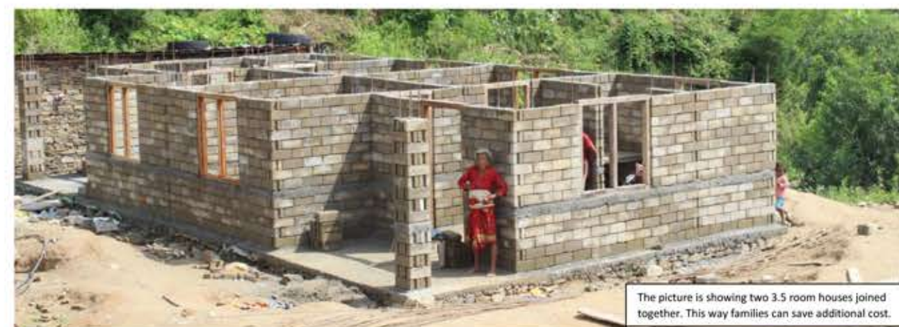
Picture 04. Two adjacent low-cost houses by Build up Nepal. Source: Build up Nepal
