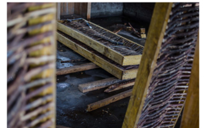
Picture 32. Interwoven wooden sticks in wood frames. Source: Photo by the Author.
