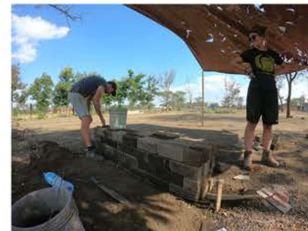
Picture 13. Interlocking bricks. Source: Photo by the Author.
