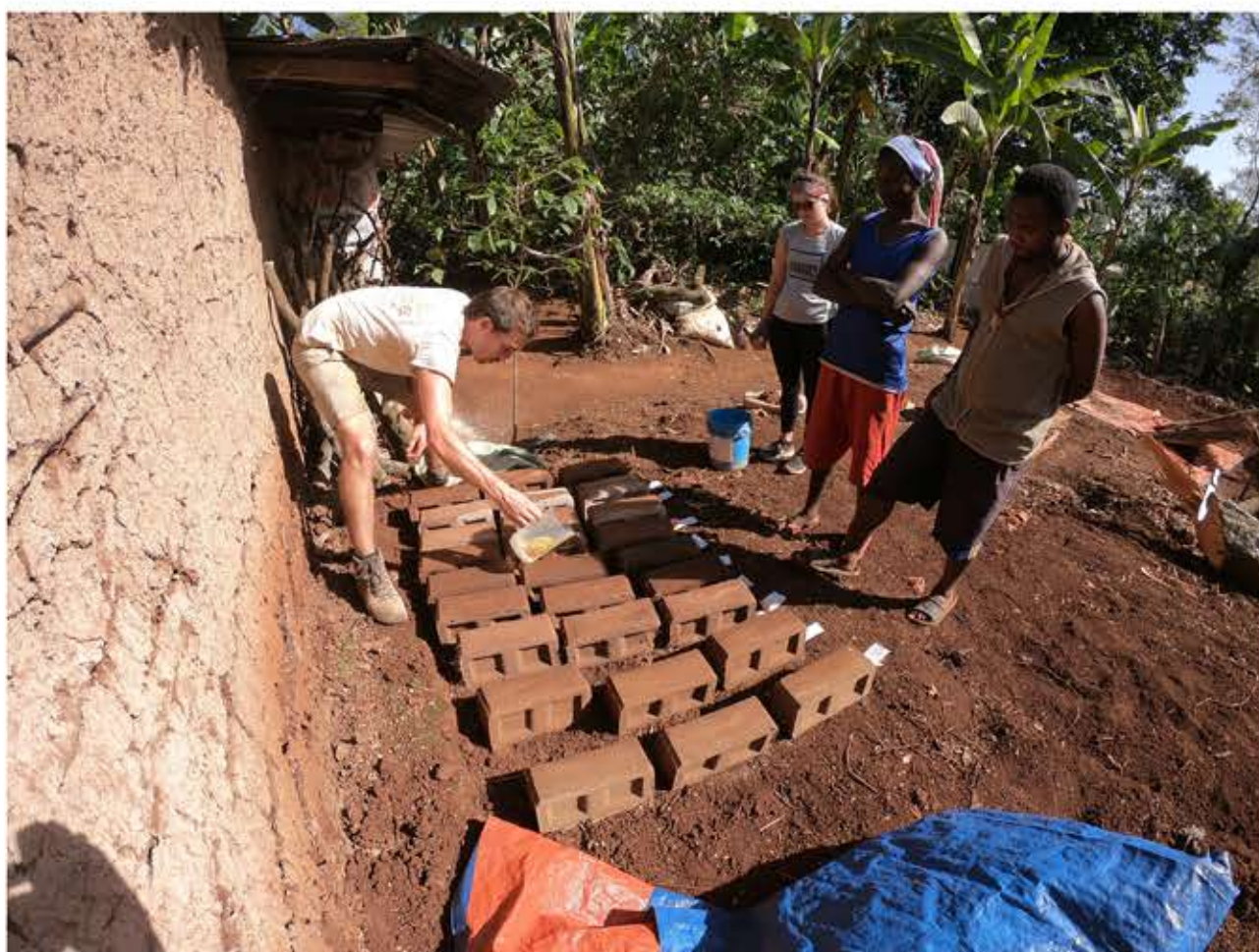
Picture 07. C-re-aid NGO intern watering the bricks. Source: Photo by the Author.
