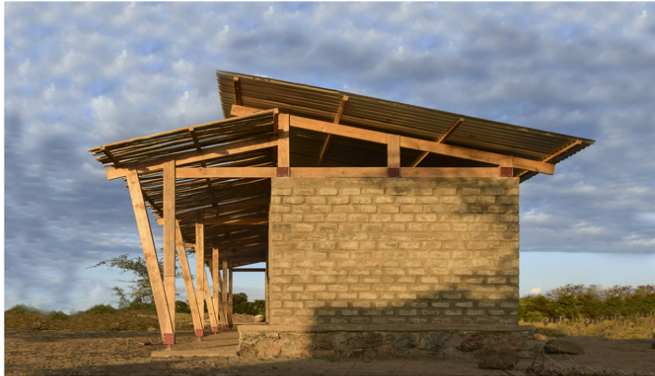
Picture 25. Doctor's house by Studio totale Firenze and C-re-aid NGO portraying roof structure, ring-beam and CEB. Source: Photo by Studio totale.
