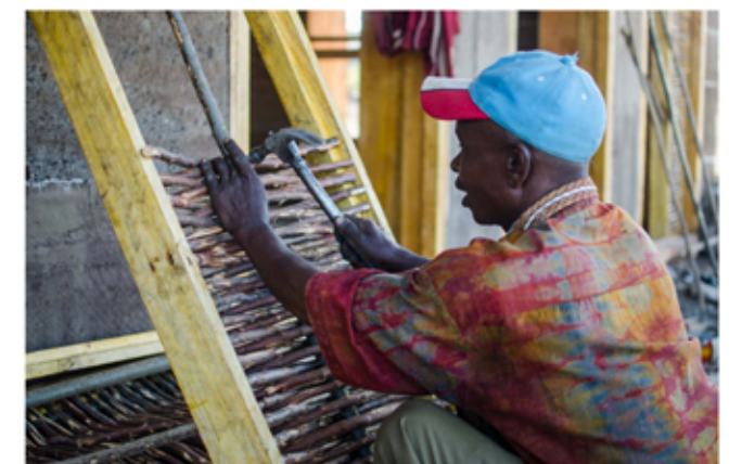
Picture 31. Tanzanian worker fixing interwoven wood sticks to wooden frame. Source: Photo by the Author.
