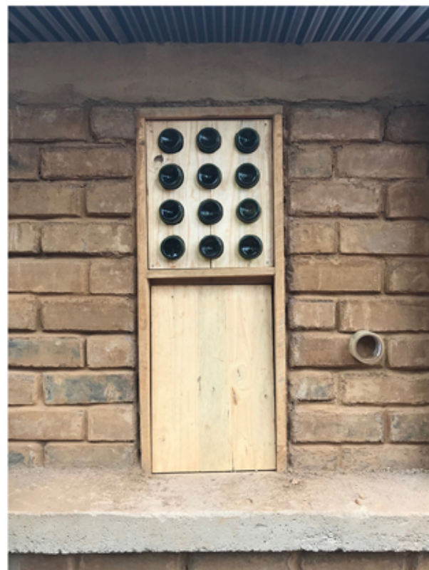
Picture 22. Back view of window prototype, developed with C-re-aid NGO, made from recycled wine bottles in wood frame. Source: Photo by the Author.
