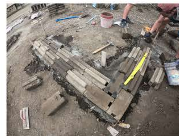
Picture 09. Interlocking bricks at corner. Source: photo by Author.
