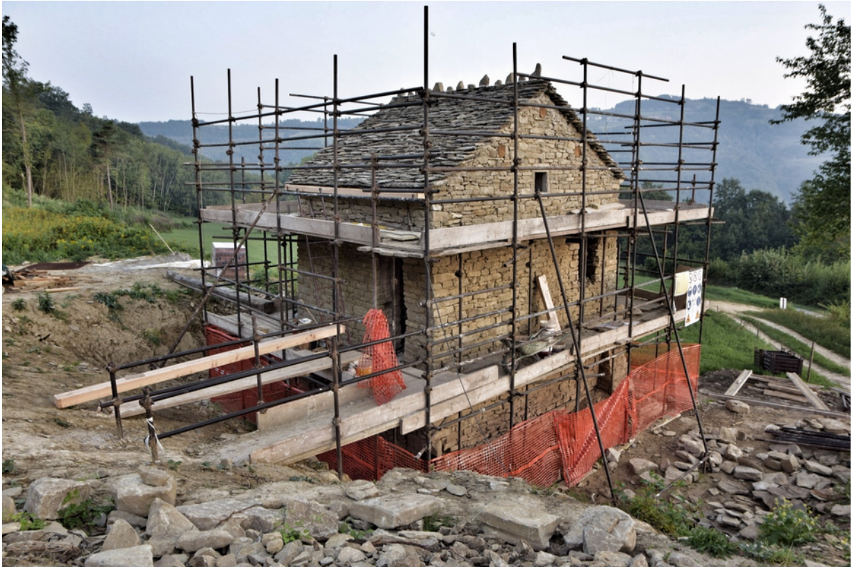
Alessandra Renzulli, The construction site , August 2018
