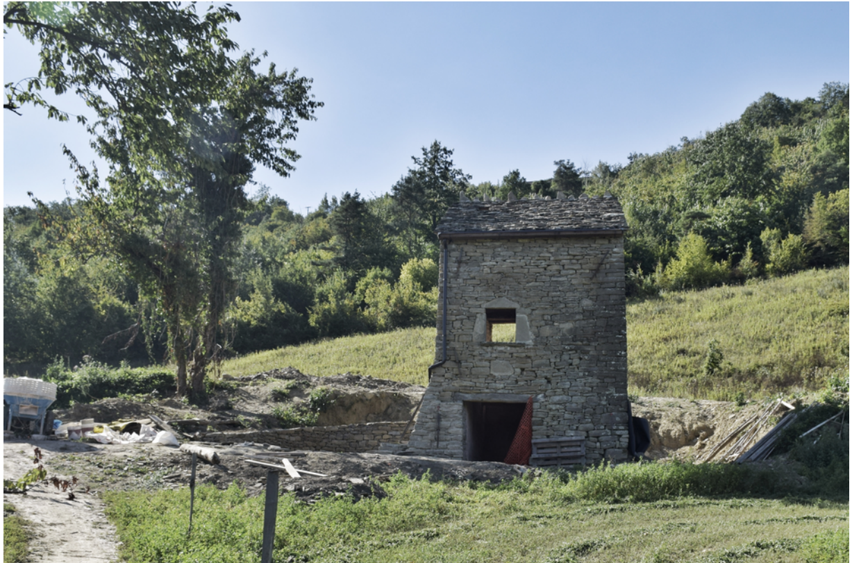
Redina Mazelli, The Lumassin after the renovation intervention of summer 2018 , September 2018
