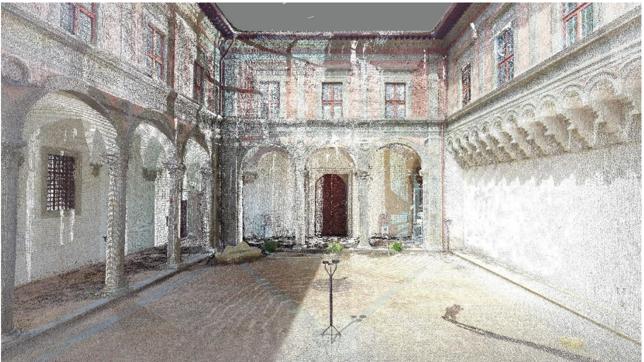
Figure 1 Point Cloud of courtyard of honor, Ducale Palace of Gubbio
