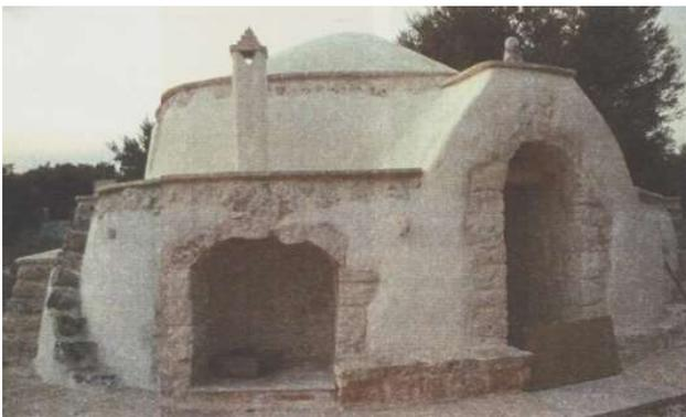
Fig. 52: Improper intervention of restoration of the 'lamia' Andriola, completed by coating the masonry with a thick layer of plaster based on cement portland. © Ilaria Pecoraro
