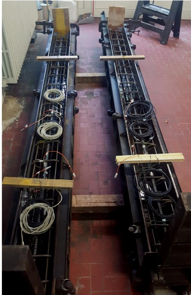
Fig. 92: Reinforcement placed inside the formworks for Beam1 and Beam2
