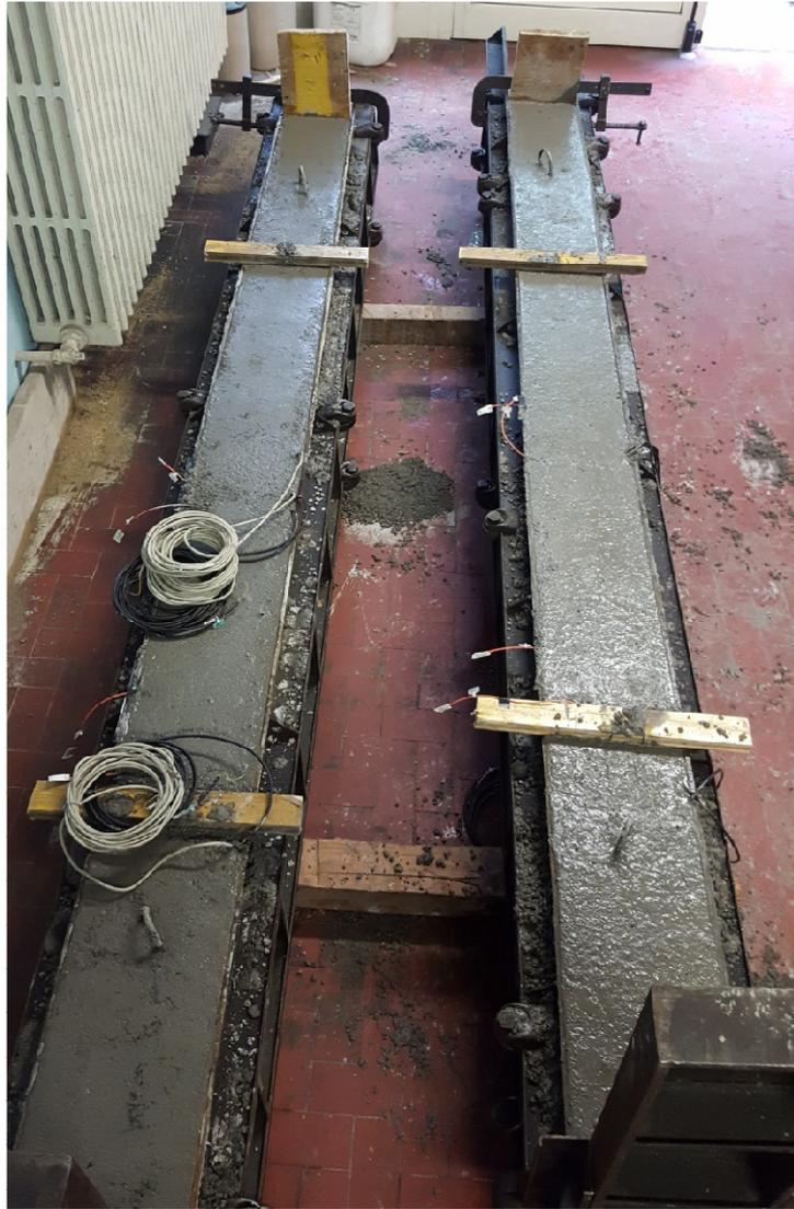
Fig. 95: Concrete poured in the formworks for Beam1 and Beam2
