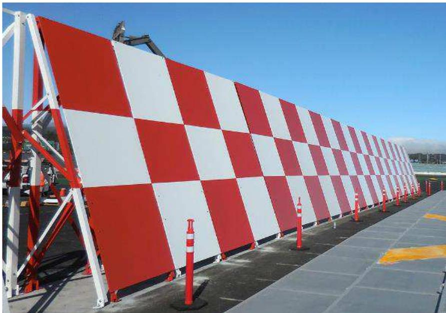
*Figura 60: barriere anti jet-blast*
