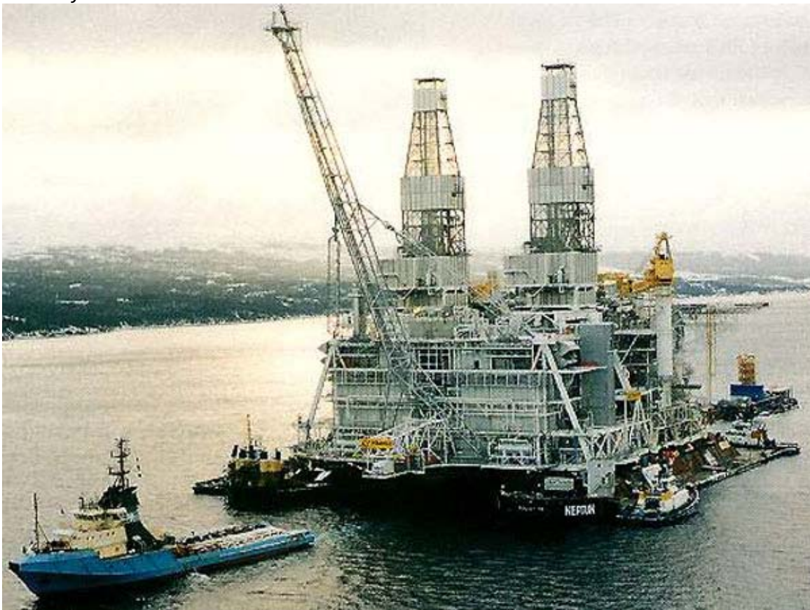
Hibernia Platform off-shore, 1990 - Grand Banks, Canada - 165.000 mc of HSC - Rck 73,8 MPa - High 111 m - Filler: silica fume - w/c 0,36
