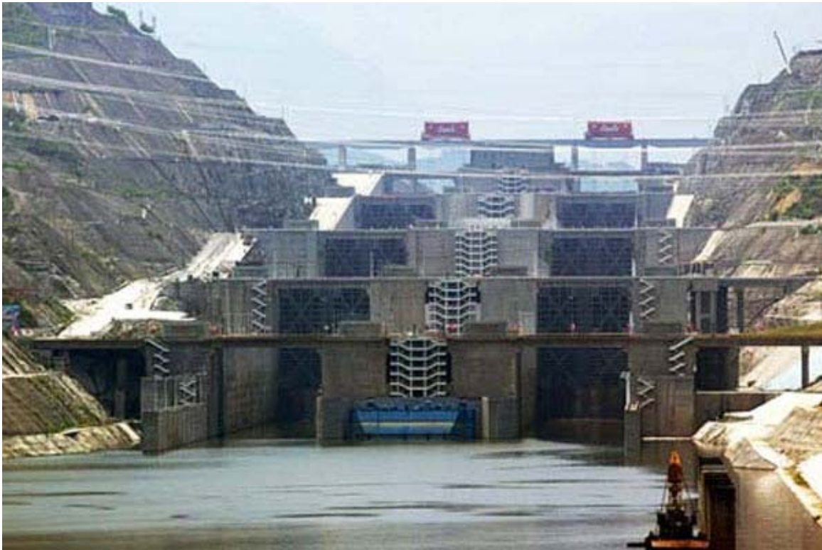
Three Gorges Dame on the Yangtze, China, under construction, 350.000 mc of HPC - Filler: fly ash
