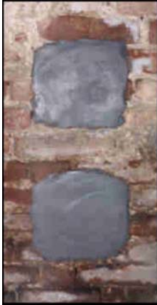
Plaster with mix of mud of granite, quicklime and fly ashes
