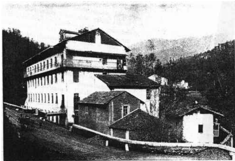
The Spinning-Mill in the oldest photograph found, showing the original aspect of the building in 1896.
