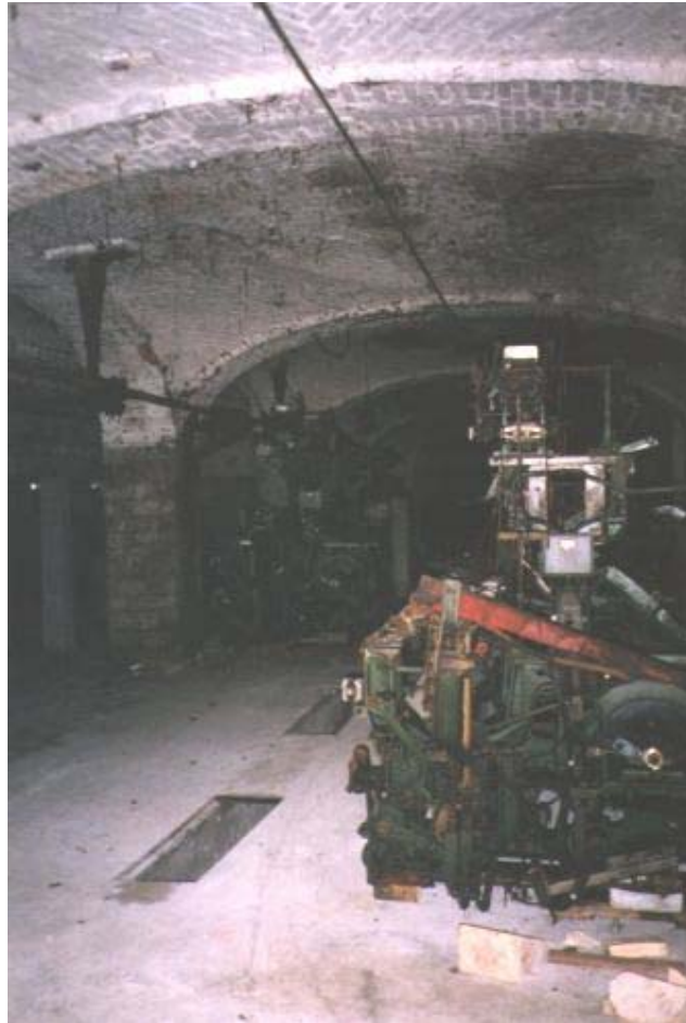
The Spinning-Mill, ground-floor workshop with pendentive dome.
