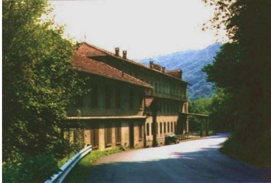
A view of the Spinning-Mill from the road facing south
