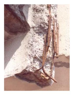
The most degradated zones are the irons of the reinforcement that are uncovered for over the 50% of their extension; the corrosion is distributed in a unvaryng way, with light localized reductions of the diameter.
