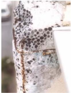
Chemical analyses were required to verify carbonation depth, and a qualitative and quantitative research on the salts present into the material.
