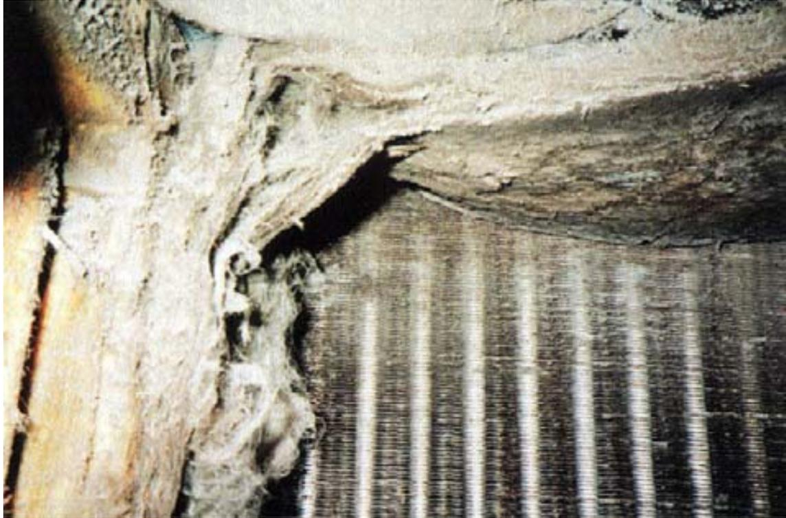
In the example the HVAC&R system is liable for a direct contamination form because of dispersion of fibrous matter from a degraded insulating coating
