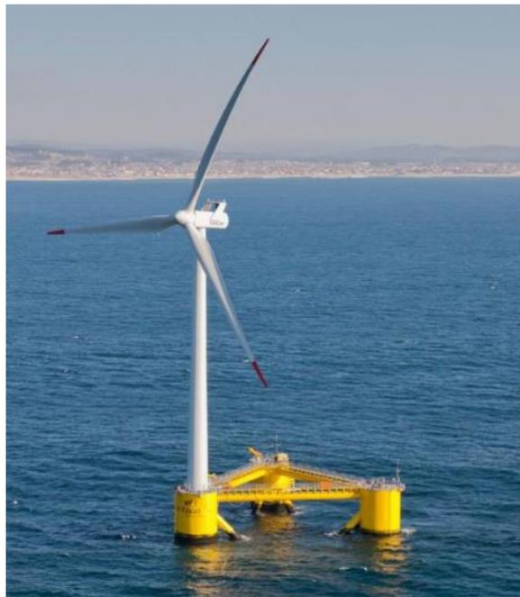
*Figure 2.6 Semi-submersible substructure concept*
