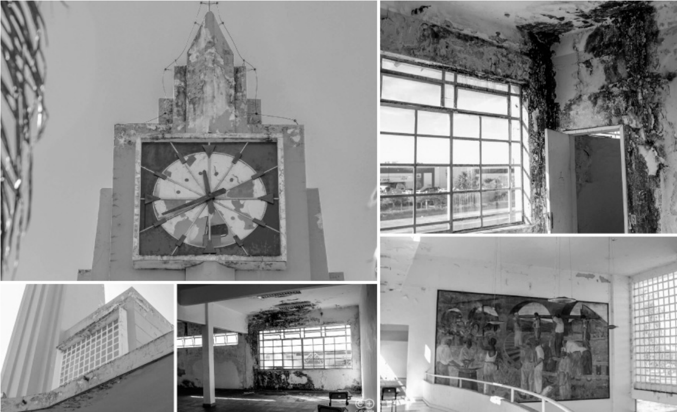
FIGURE 27 - Set of images of the former Railway Station Building previously its restoration project showing its decay problems.
