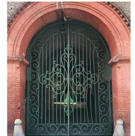
Fig 90: Handmade wrought iron entrance door.
