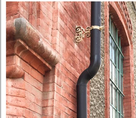
Fig 89: Ornamental bracket connecting the downpipe to the pillar.
