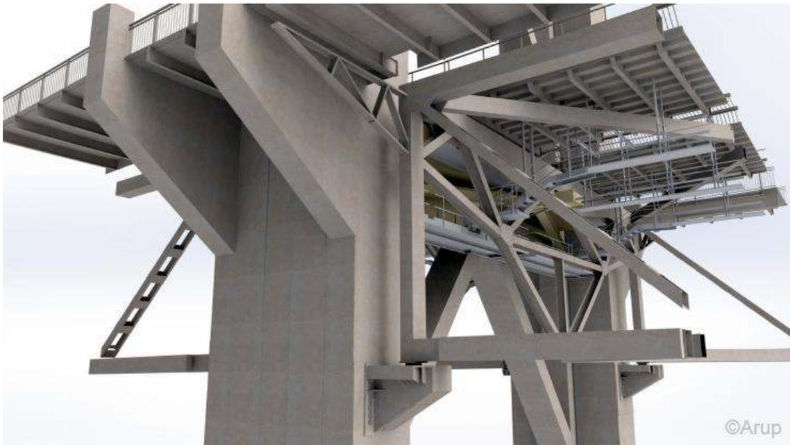
*Figure 3.7: New sliding bearing (Arndt M., 2017)*
