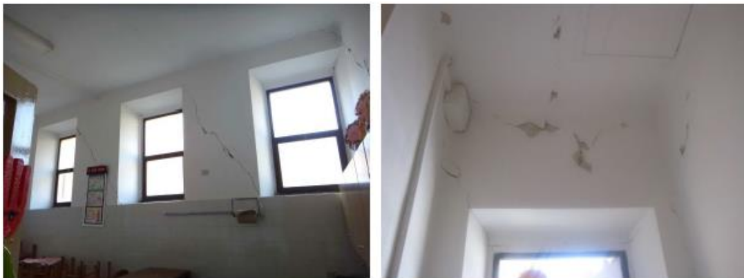
Figure 0.1: State of damage within the structure following the event of 24 August [16].
