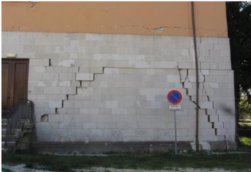
Figure 0.7: Shear-sliding Lesions in the Northwest wing at the cantonal male [16].
