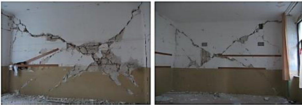
Figure 0.6: Shear injuries for diagonal cracking in the males of the body A oriented Y-direction [16].
