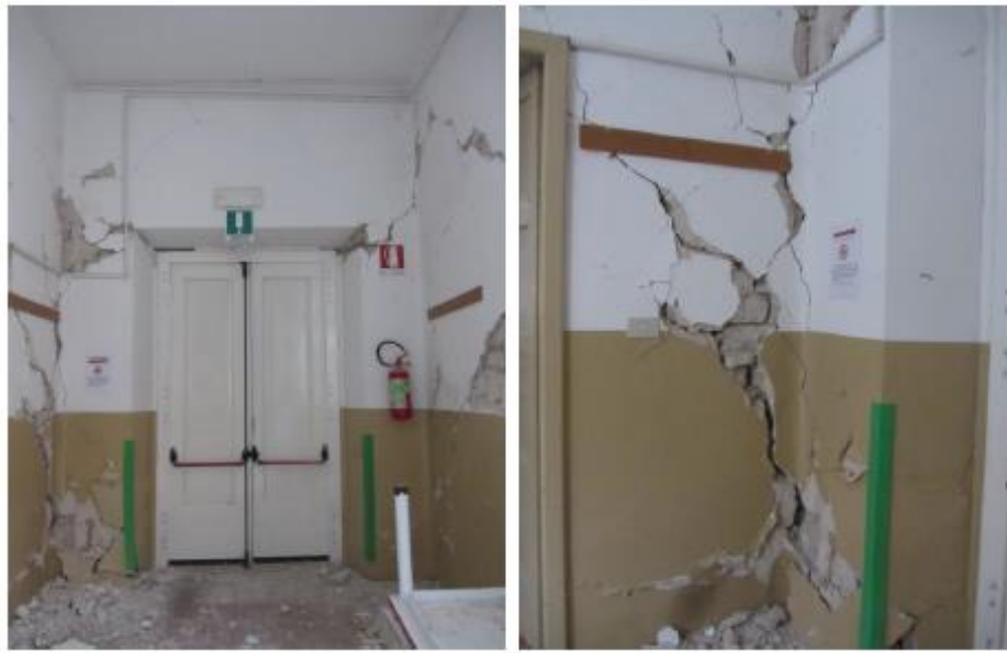
Figure 0.8: Internal vision with severe pseudo-vertical lesions in the North-west wing [16].
