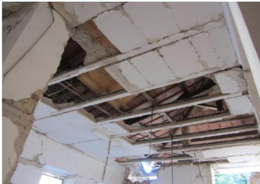
Figure 0.11: Extended Collapse of the attic floor [16].
