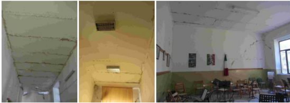
Figure 0.3: Minor sub-horizontal lesions to the interface with the internal masonry on the first floor [15].
