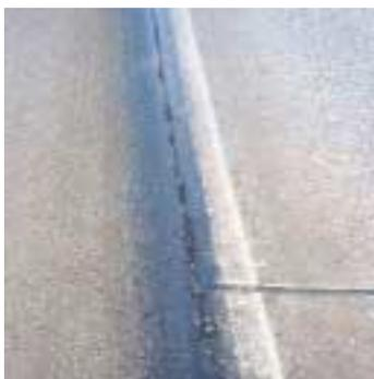
FIGURA 41 - DISTACCO DELLA CORSIA RISPETTO ALLA BANCHINA
