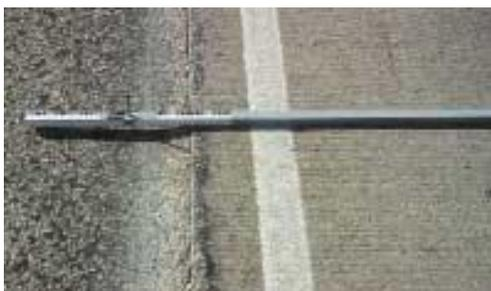
FIGURA 40 - CADUTA DELLA CORSIA RISPETTO ALLA BANCHINA
