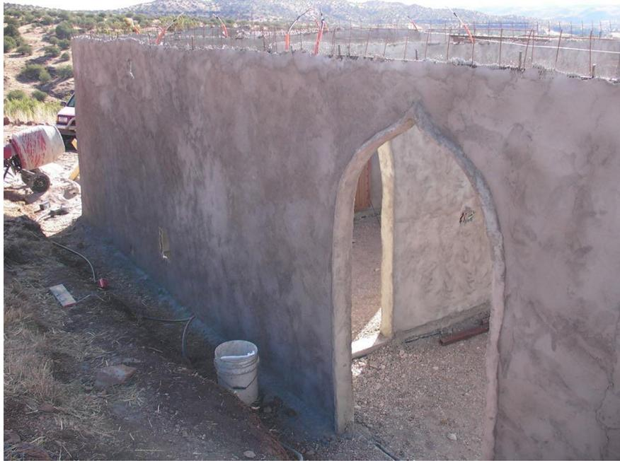
**Figure5. 11:** Ferro-cement wall of a House
