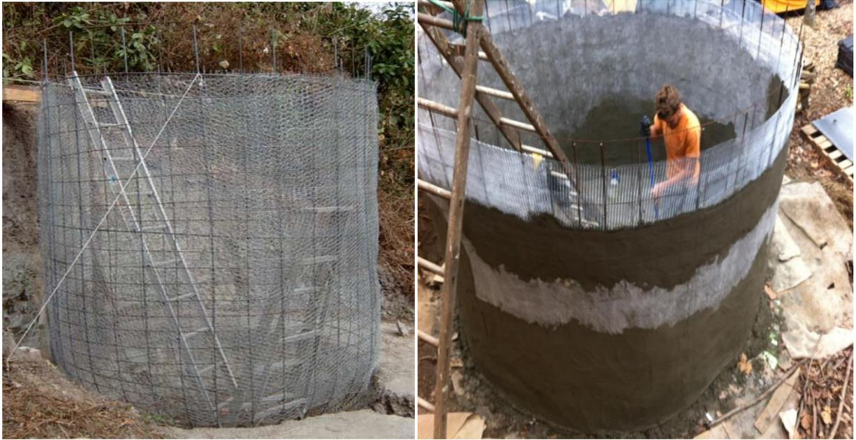
**Figure5. 8:** Water tank with rounded reinforced wall
