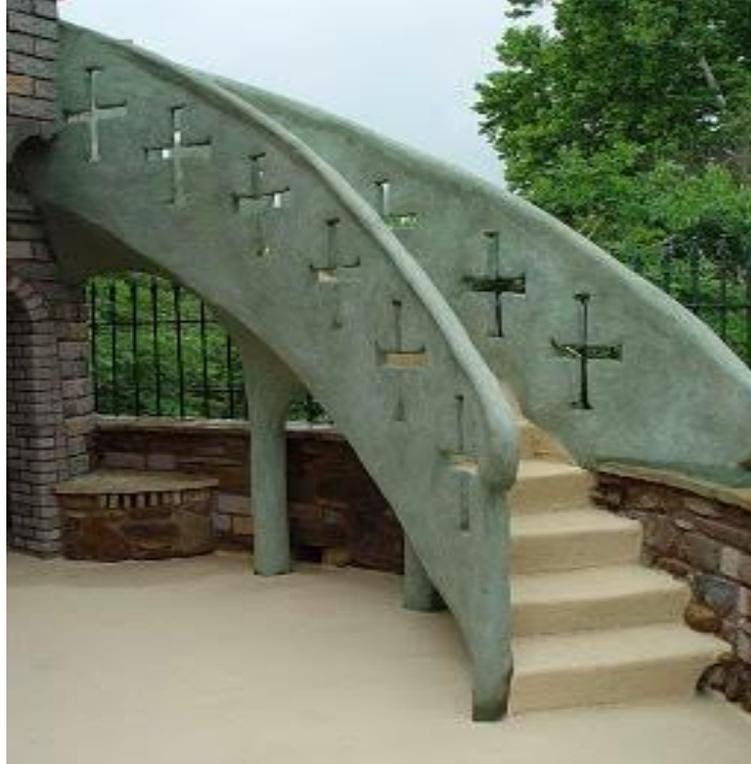
**Figure5. 17:** Ferro-cement stairs case
